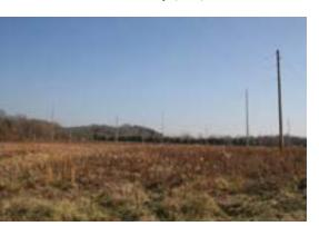
Not a power line installation but a big time Rhombic array antenna at WWCR's antenna farm. This, along with its 100 kW transmitter, accounts for its needle bending signal strength across North America. Look for plenty of real estate if you plan this type of antenna for your own HF broadcast station. (Photo by Cameron Keel courtesy WWCR)
